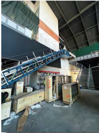
Baylor Escalator before Cladding
